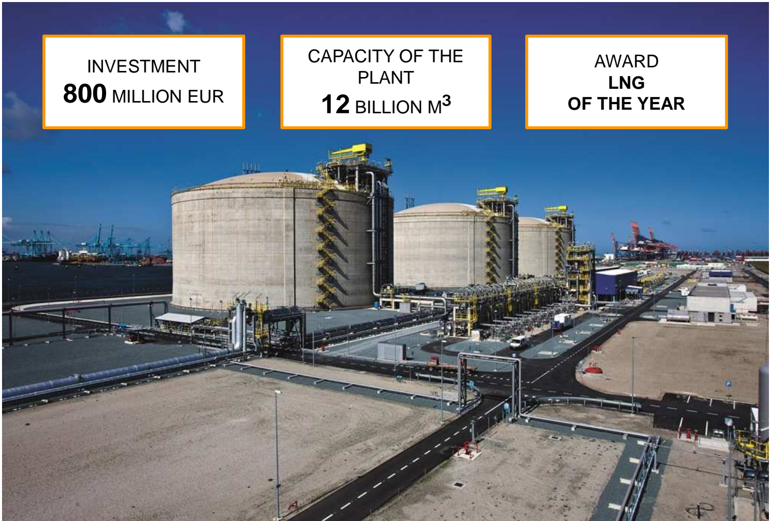
Three storage tanks of 180.000 m 3
